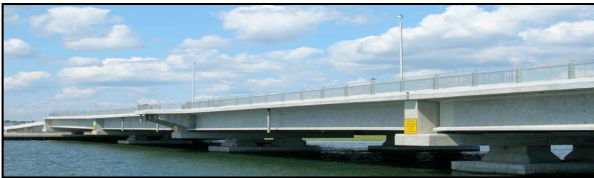
Newly constructed bridge over Elbow Thorofare (Contract A)
