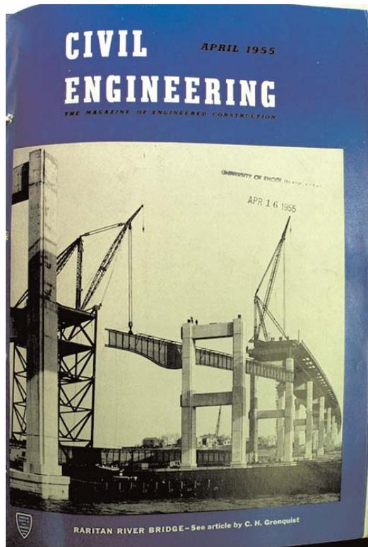
*Specially built to be easily widened to meet future traffic demands, the Driscoll Bridge was cited for its progressive design and was featured on the cover of the April 1955 Civil Engineering magazine. Shown is the lifting of the massive 263' main girder, weighing over 200 tons, fabricated and erected by the Bethlehem Steel Company.*
