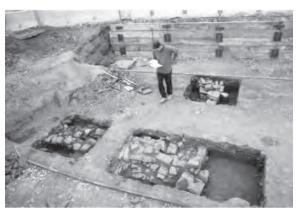
hurricane that flooded the property in 1749 left clay caked to the bottom of the house foundations, and the drainage ditch was clogged with silty clay mixed with brick fragments. Flatt rebuilt the house, placing new cut stones on top of the old ones. Only the southeast corner of the foundation was uncovered archaeologically, but it suggested a substantial structure,
