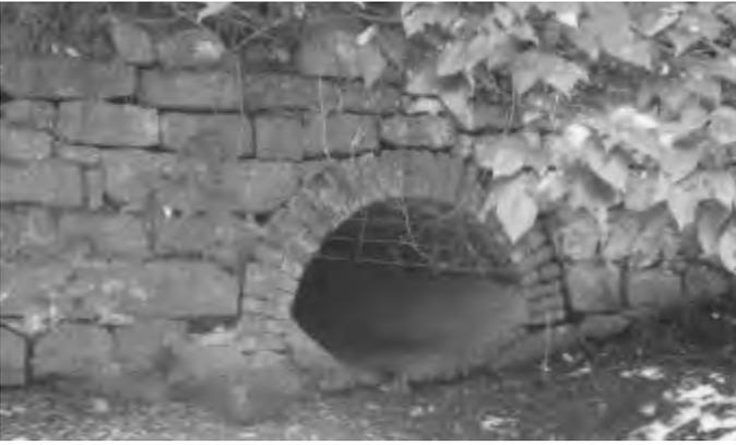
*This masonry culvert, near the Route 130 bridges, carried the railroad across a small stream [Source: Hunter Research, Inc.].*
